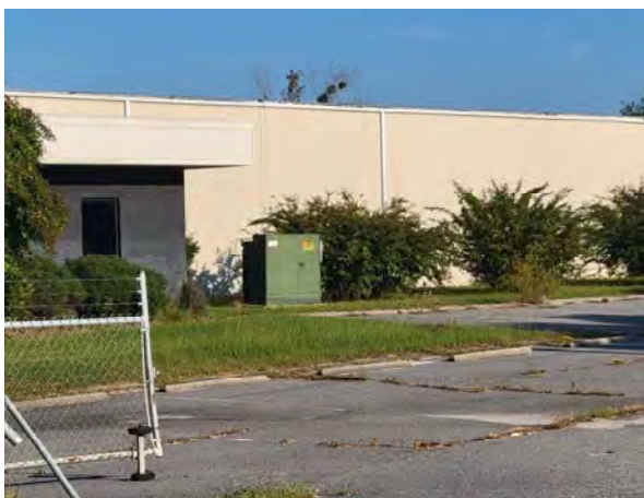
Representative view of pad-mounted transformer observed adjacent to the Site within the Titan Flow Control, Inc. property.
