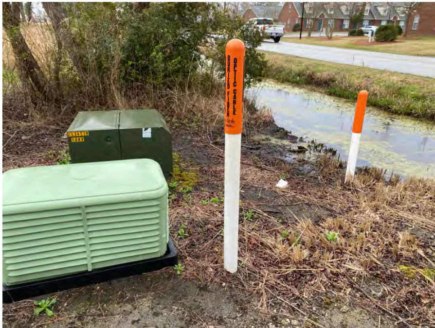
Photo 22: Pipeline markets and pad-mounted transformer on subject property.
