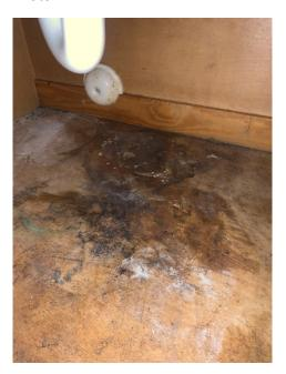
Suspect visible mold growth in the kitchen cabinet underneath the sink
