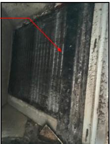
Dust and debris noted on the HVAC return vent.
