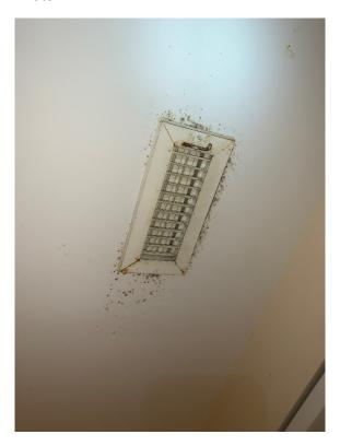
Suspect visible mold growth around the HVAC supply vent in the 2<sup>nd</sup> floor hallway
