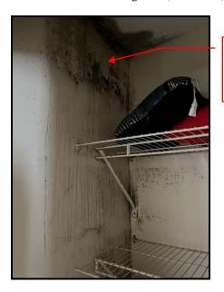
Suspect visible mold noted on the rear closet wall and adjacent ceiling.
