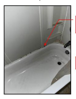
Suspect visible mold noted on the bathtub edges.
