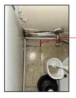
Exposed wood subfloor noted by the water damaged wall and base.
