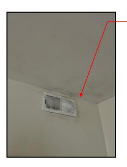
Suspect visible mold on diffuser, wall and ceiling at rear left of living room.
