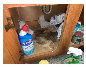
Apparent water damage/suspect visible mold growth in the bathroom cabinet with sink.
