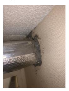
Suspect visible mold growth above the front left bedroom door frame.
