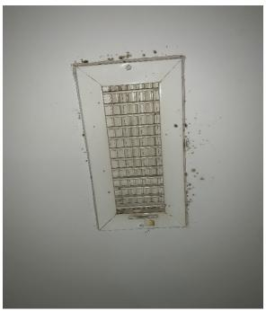
Suspect visible mold growth around the HVAC supply vents in the  $2^{nd}$  floor rear right bedroom Photo 5
