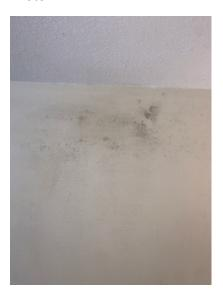
Suspect visible mold growth on the front left bedroom wall over the bed.
