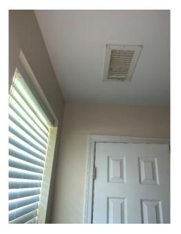
Suspect visible mold growth/dust on the HVAC supply vent in the front right bedroom.
