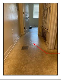
Water staining noted under an HVAC supply diffuser.
