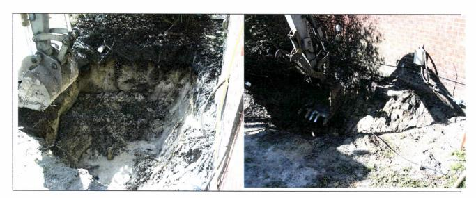
Photos showing the final "foot print" of the contaminated soil excavation.
