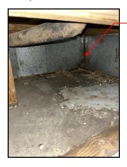
Excessive dust/debris and suspect visible mold in return plenum.
