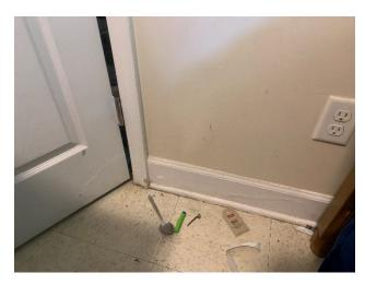
Apparent water damage on the rear left bedroom rear baseboards and closet door.
