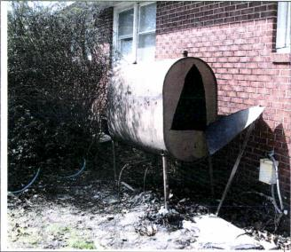
The aboveground oil tank was standing very close to the back of the house. This picture shows the tank cut open to allow interior cleaning.
