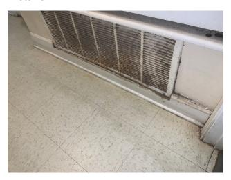
Apparent water damage on the hallway front baseboard adjacent to the bedroom associated with air handler/washer heater closet.
