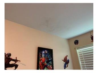
Apparent water damage/suspect visible mold growth on the rear left bedroom ceiling.
