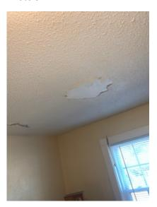
Apparent water damage on the front left bedroom plaster ceiling.
