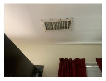
Suspect visible mold growth/rust and condensation on the HVAC supply vent in the living room near the front exterior door.
