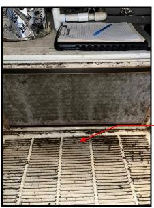
Dust and debris noted on the HVAC evaporator coils.
