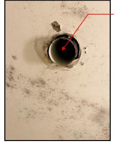
Missing HVAC supply diffuser/boot.
