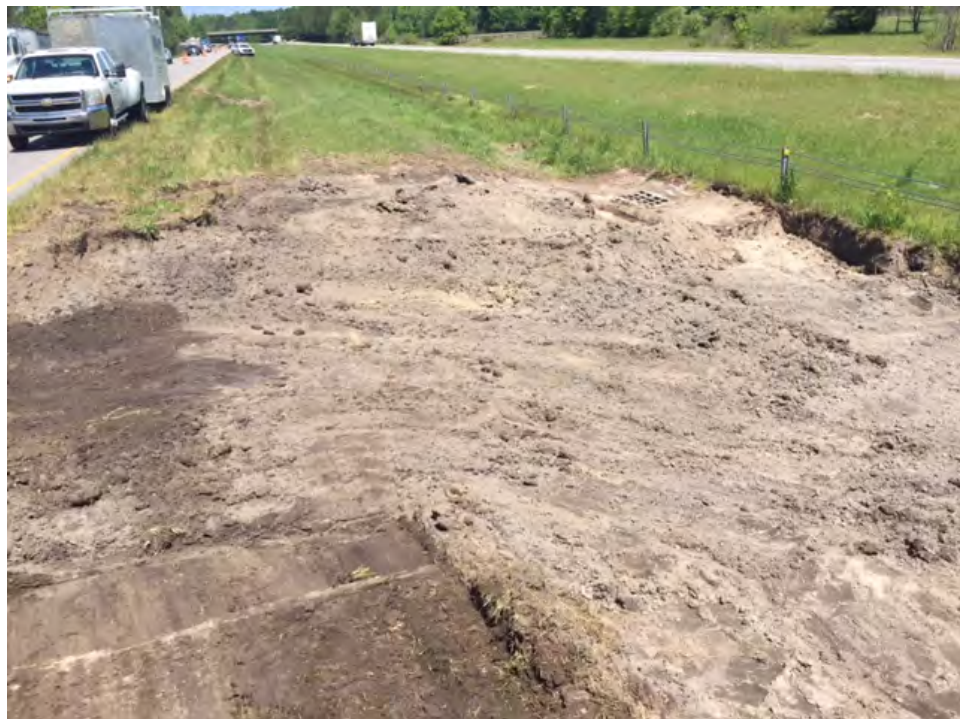
Highway median remedial excavation
