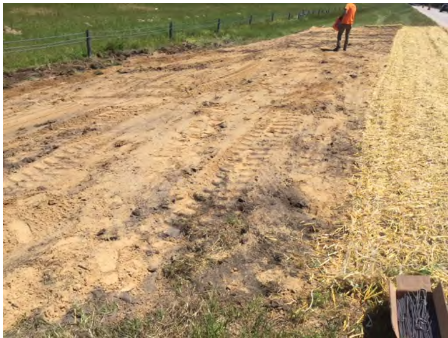
Center median backfilled with strawing in progress
