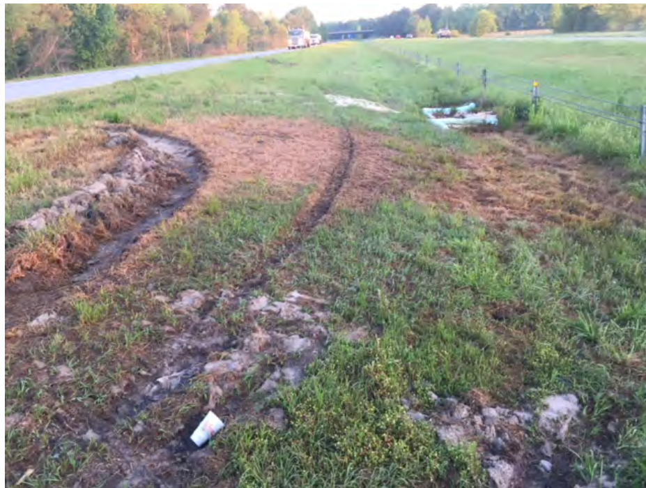
Ruts with fuel and booms around catch basin in highway median
