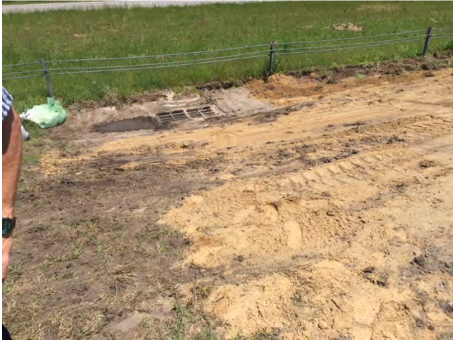
Center median backfilled
