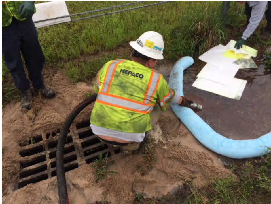
Sand berm and ponded liquids outside of catch basin
