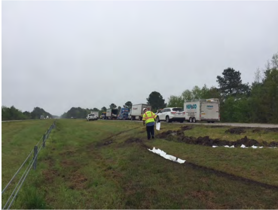
Placement of sorbent pads to collect liquids
