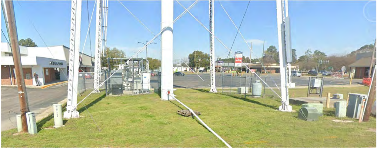
Water Tower by Pembroke Drug, 205 W 3rd St, Pembroke, NC 28372
