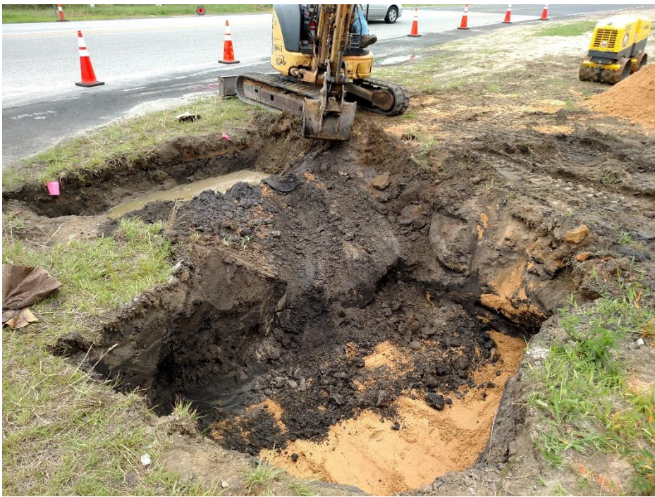
Photo #7: A view of the UST excavation prior to backfilling activities.
