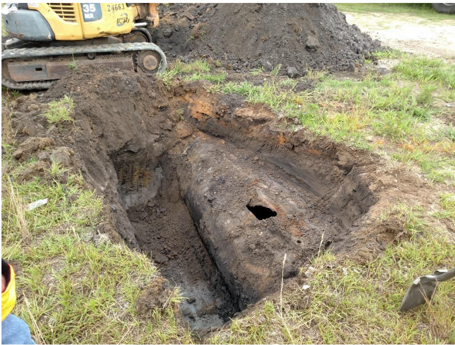
Photo #3: A view of UST-2 subsequent to being exposed.
