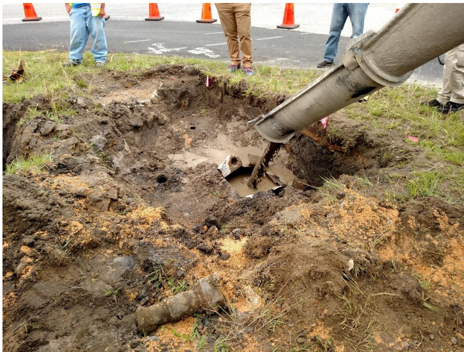
Photo #6: A view of flowable fill placement and in-place closure of UST-1, facing west.
