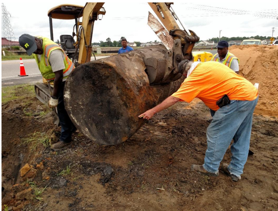
Photo #4: A view of UST-2 following removal
