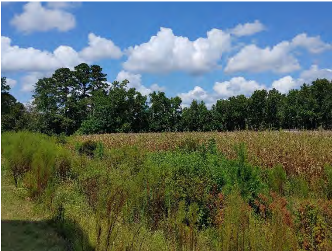
9: View of overgrown drainage ditch along southwestern boundary of property.
