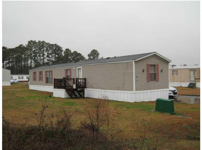
Mobile home community north from the Subject site
