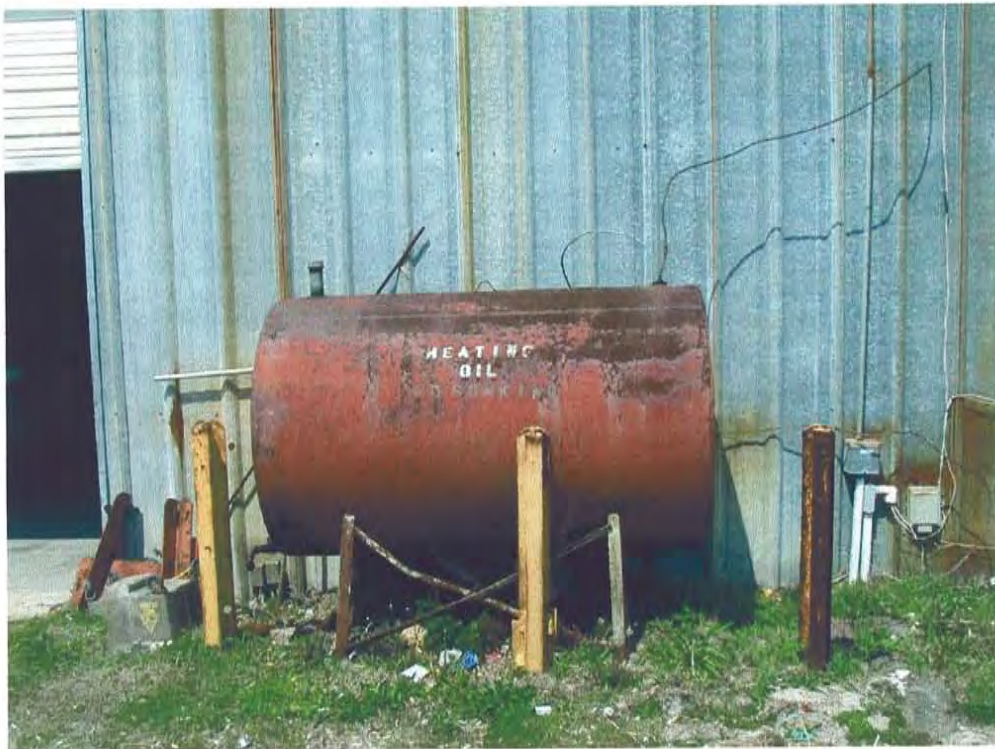
Photograph No. 2: One of two heating oil aboveground storage tanks used by the maintenance garage, which is located on the site.
