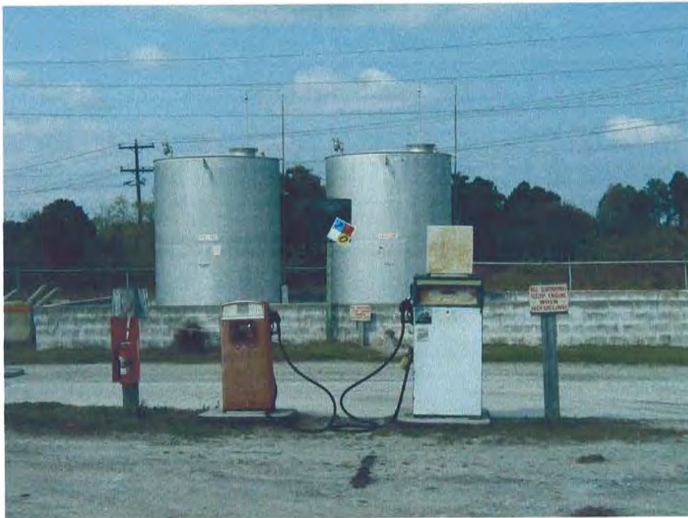
Photograph No. 3: Two 4,000-gallon above ground storage tanks, and associated pump islands, used to store gasoline and diesel fuel on the site.
