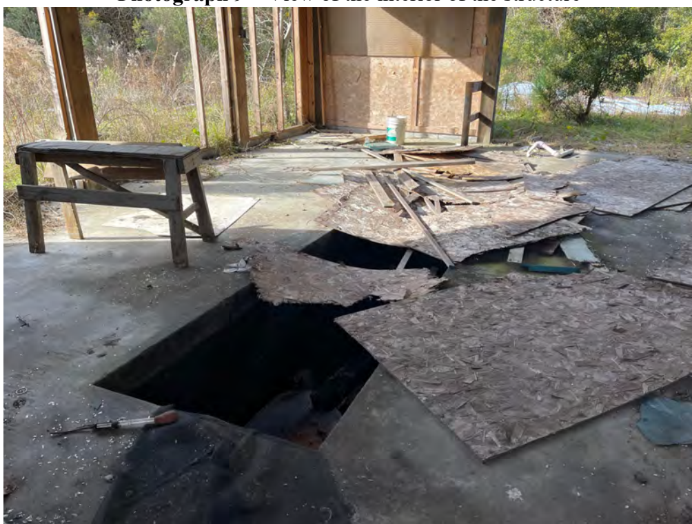
Photograph 10 – Concrete sub grade maintenance pit
