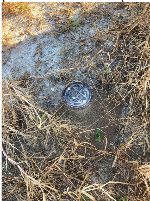
Photograph 6 – Water cleanout on southeastern portion of the site
